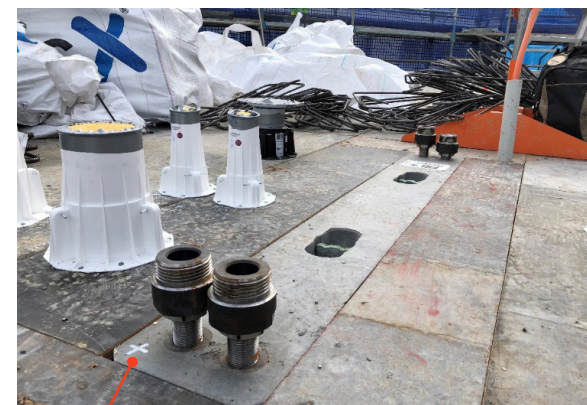
Mark to indicate which coupler is set to level – the "RL" coupler
