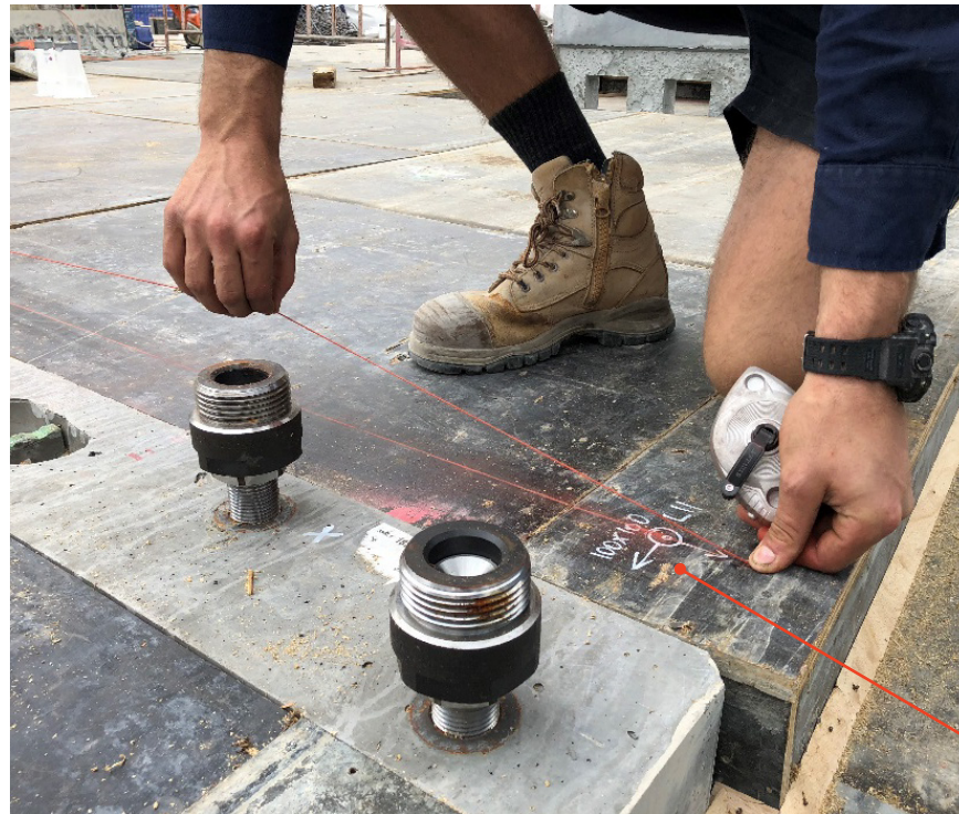
Offsets marked by the site surveyor.
